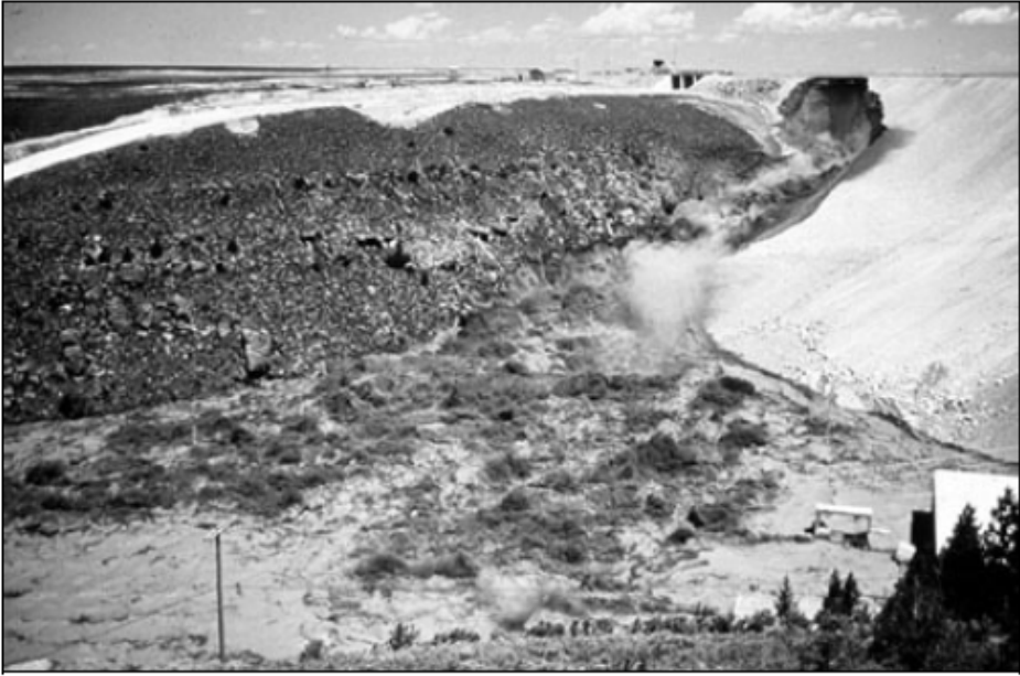
Figure 2-8. Teton Dam Failure Sequence, Beginning of Final Failure. Source: Independent Panel (1976).
