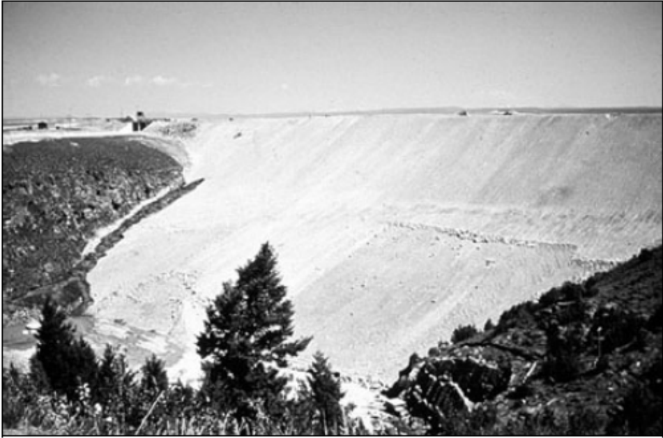
Figure 2-6. Teton Dam Failure Sequence, Initial Erosion.
