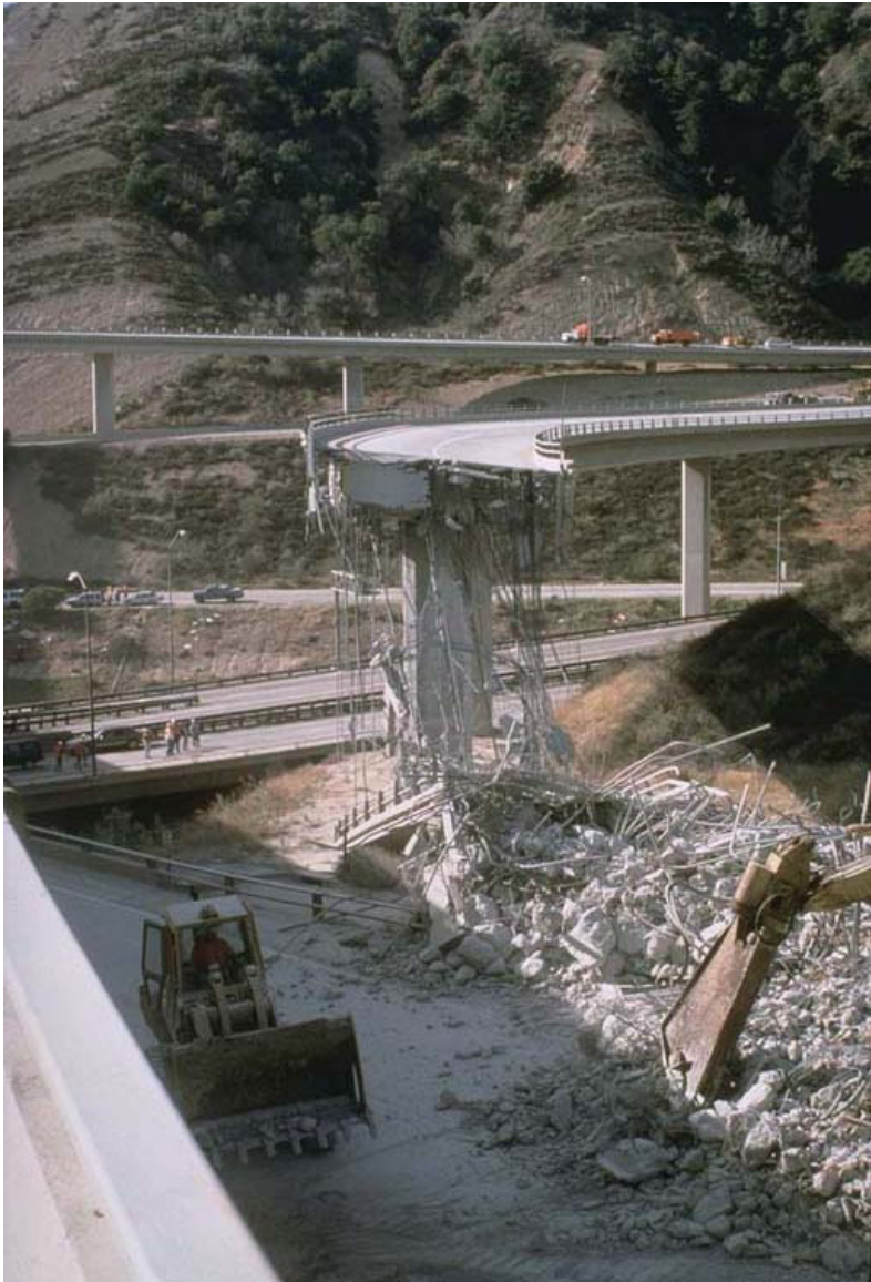
Figure 4-1. Antelope Valley – Interstate 5 Freeway Interchange Failure – 1994. Source: J. Dewey, USGS.
