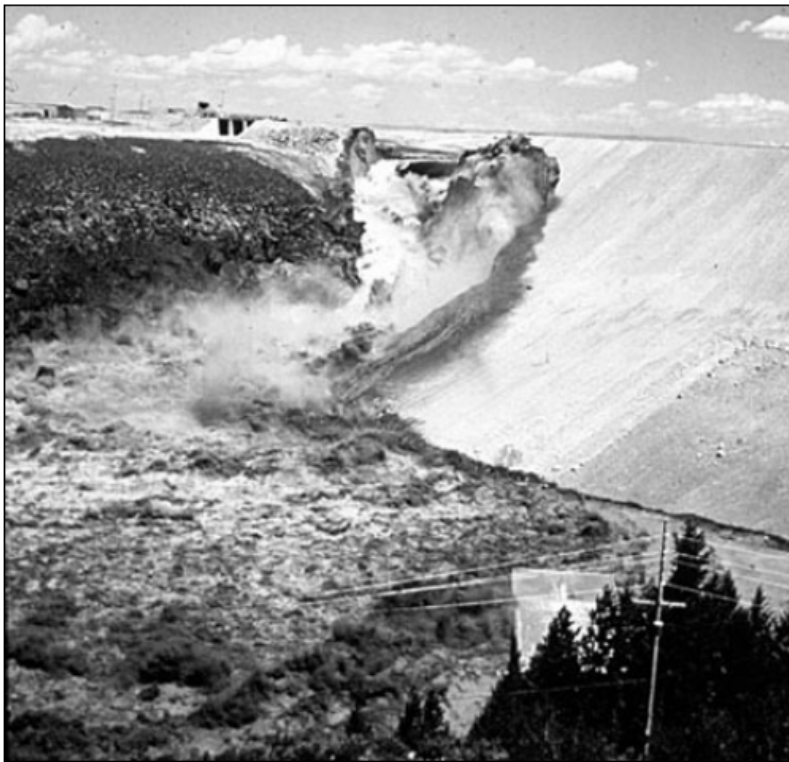
Figure 2-9. Teton Dam Failure Sequence, Failure of the Dam. Source: Independent Panel (1976).
